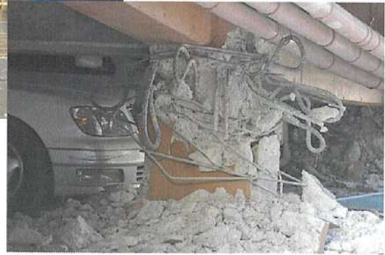
Pilotis style 7-story RC construction condominium The pillar on the first floor buckled (1-chome, Demachi, Nishi-ku, Kumamoto City) No noticeable damage to the temple gate directly next to it
