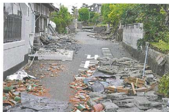
Concrete block walls collapsed everywhere and scattered across roads
