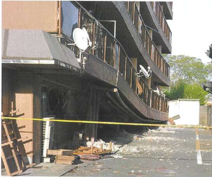
Pilotis style 7-story RC construction condominium The pillar on the first floor buckled (1-chome, Demachi, Nishi-ku, Kumamoto City) No noticeable damage to the temple gate directly next to it
