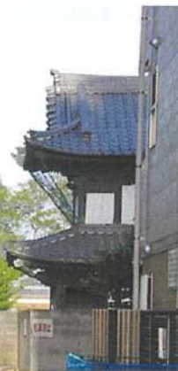
The temple gate on the right remained almost undamaged; only a part of the white wall peeled off.
