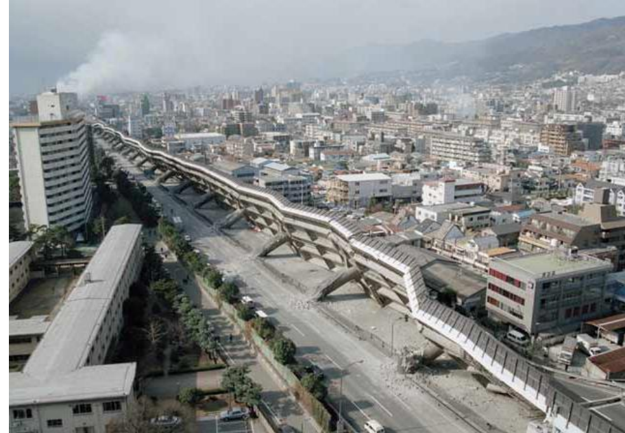
Hanshin Expressway (Photo: Kobe City)
