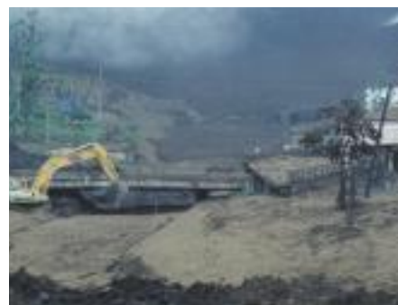
Restoration Work at Mt.Usu under Remote Control
